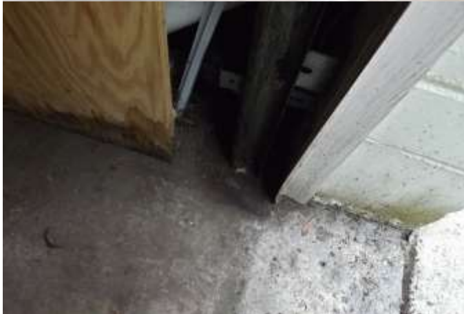
Garage safety beams in good working condition
