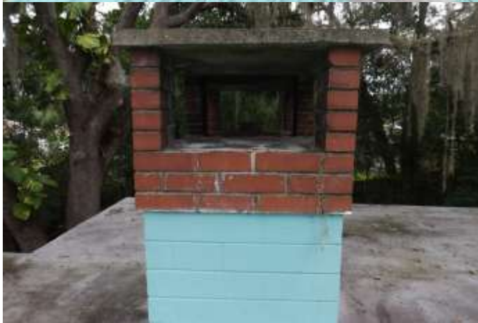
Spark arrestor not present (Recommended)
