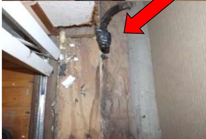
installed in junction box with cover.
