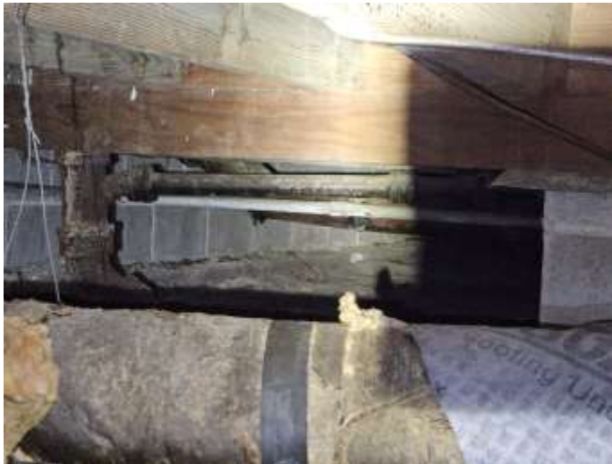
Drain Cast Iron
