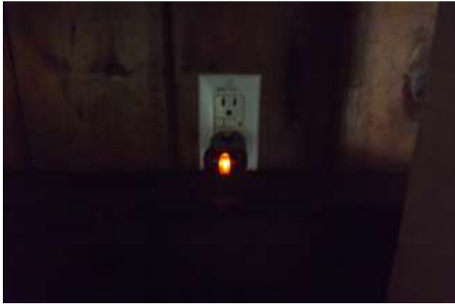
Open Ground /GFCI Protected
