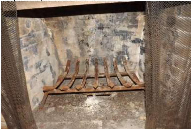
Damper missing & Corrosion visible
