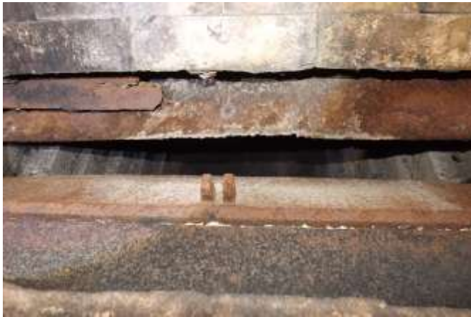
Damper missing & Corrosion visible
