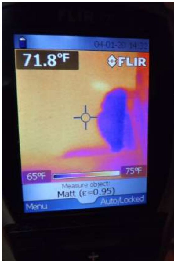
Infrared camera moisture damaged wall & Floor Repair
