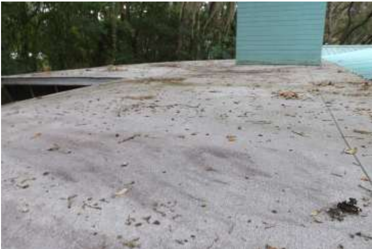
Flat roof Roof Adhered Modified Membrane
