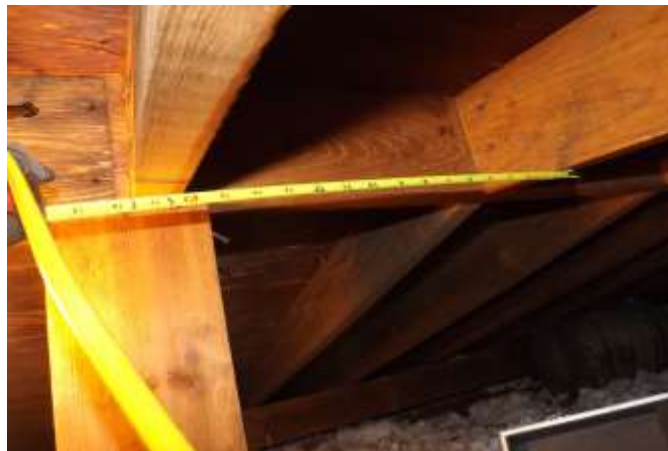
Rafters 16 inches spacing
