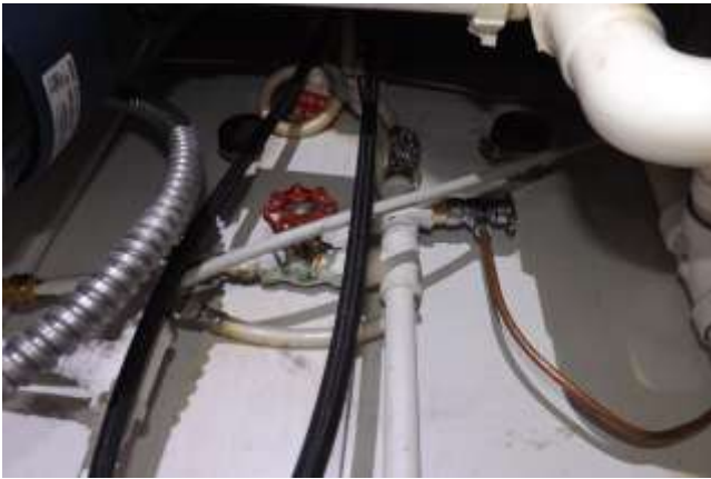
Kitchen/ hot water pipe copper/Cold water pipe galvanizes
