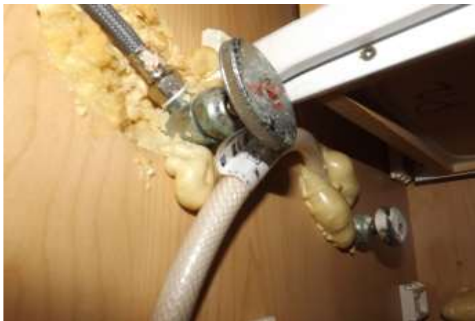
Shutoff handle appears to be crack replacement needed - Water pipes not visible
