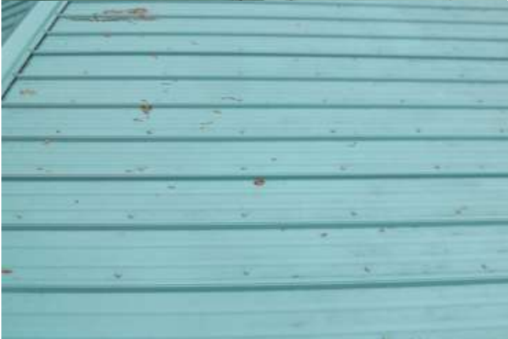
Roof screw life expectancy 15 to 25 years plan budget
