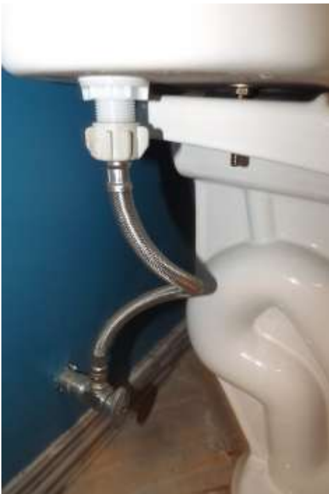
Hall Toilet Water Pipes not visible
