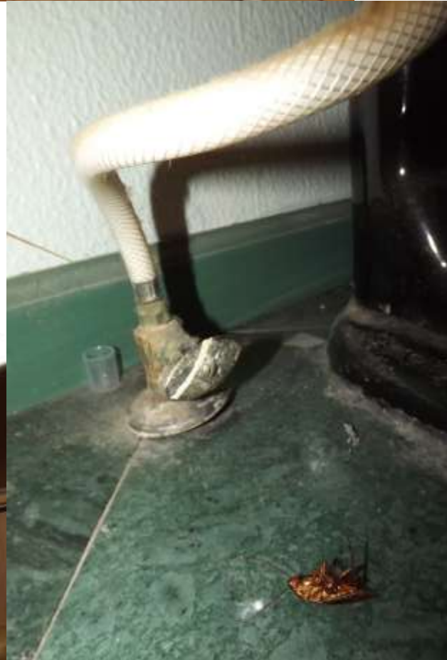
Shutoff handle appears to be crack replacement needed - Water pipes not visible
