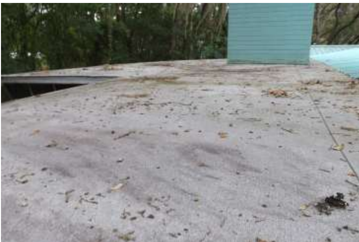
Flat roof Roof Adhered Modified Membrane
