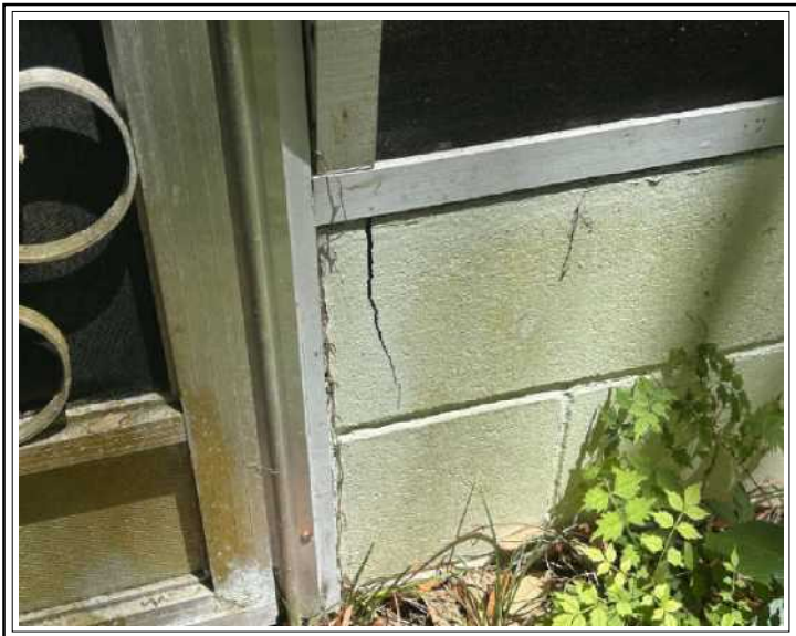
SEAL CRACKS
