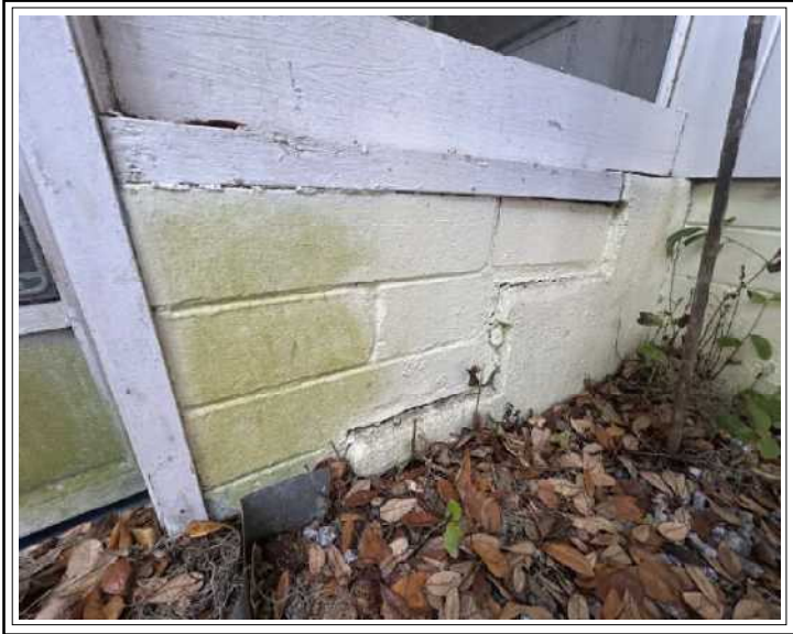
PRESSURE CLEAN / PAINT / SEAL CRACKS
